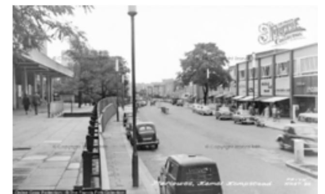
The new town centre in 1960s
